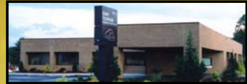
A Telecommunications Provider
